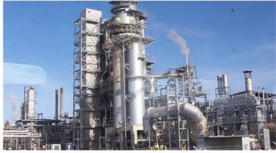
Dangote Refinery Commissioned – May 22 nd
